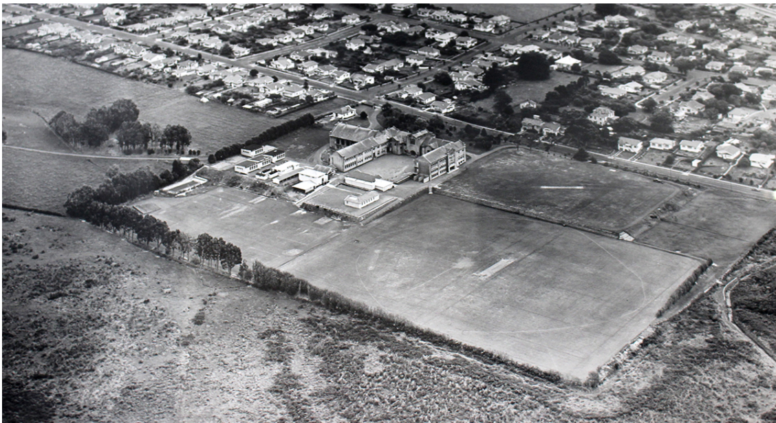
An aerial view of the school in 1949.
